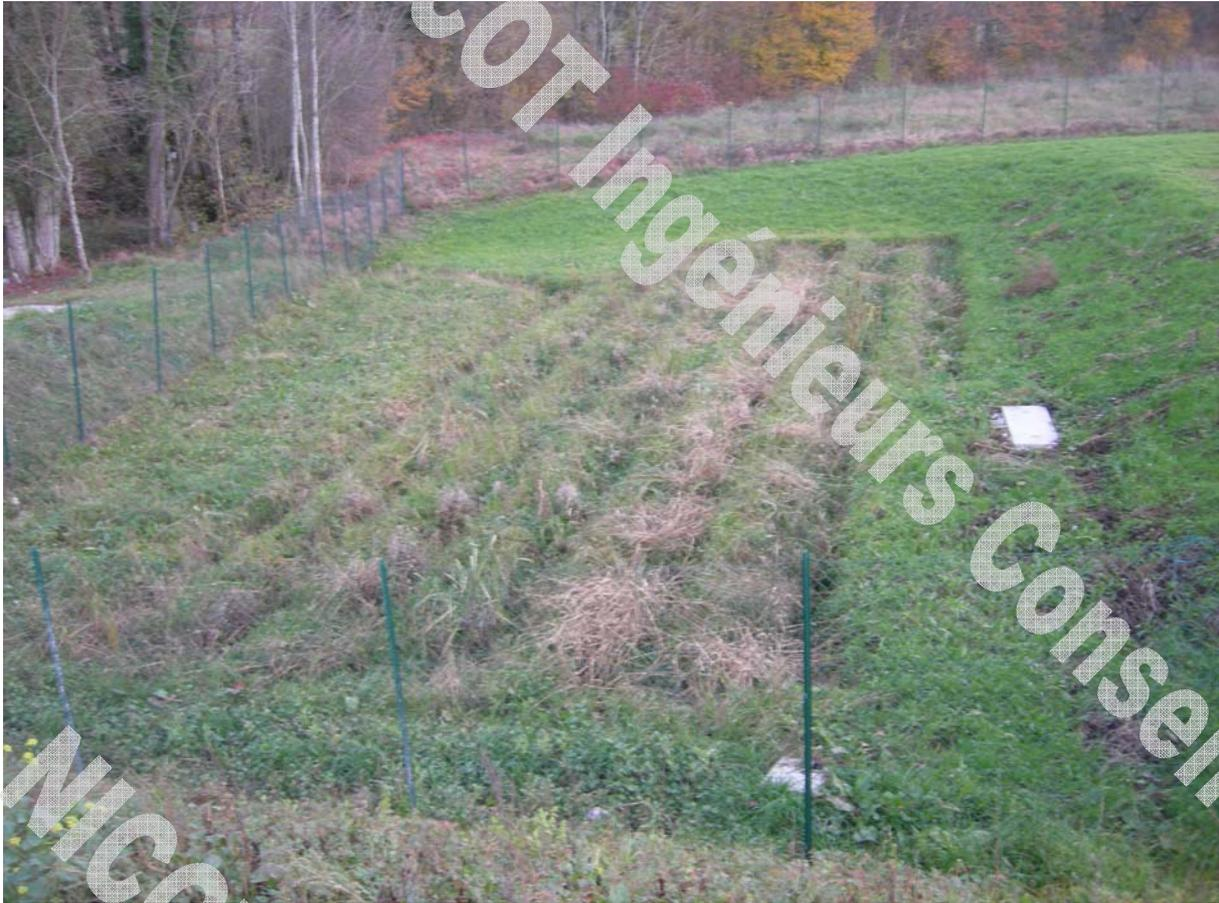
**EXEMPLE DE TRAITEMENT TERTIAIRE PAR DISSIPATION APRES LA STEP DE SAVIGNY**
